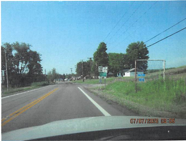
23. State Route 9 (First Street)
