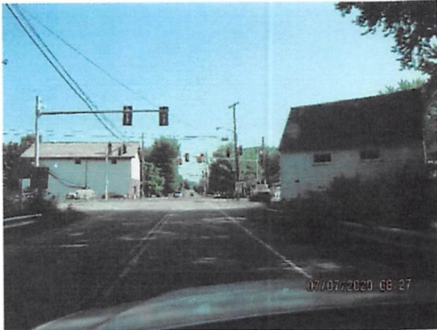
11. Route 9 & Route 30 Intersection
