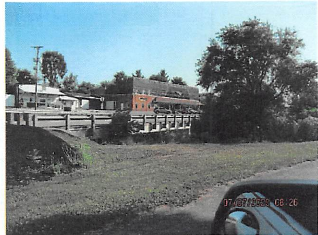
14. Route 30 Stream Crossing
