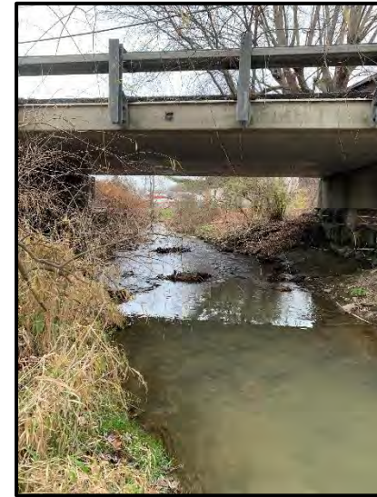
Photo 30: STREAM-2SP location, crossing under bridge carrying 1 st Street, facing west.
