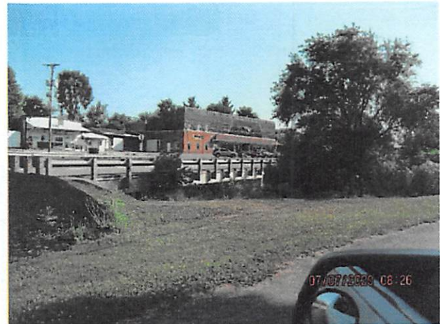
14. Route 30 Stream Crossing
