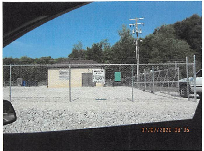
24. Kensington Treatment Plant
