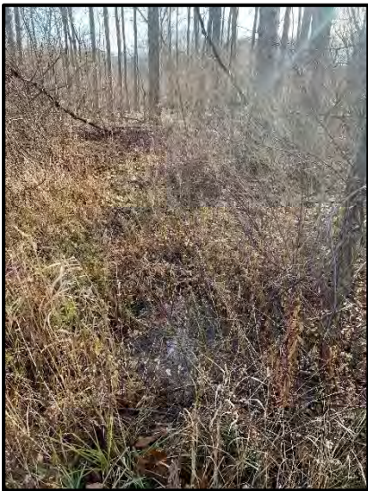
Photo 15: 11/24/2020 – Standing water observed near WET-4SP, facing south.
