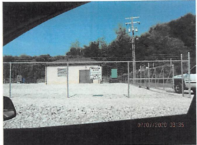
24. Kensington Treatment Plant
